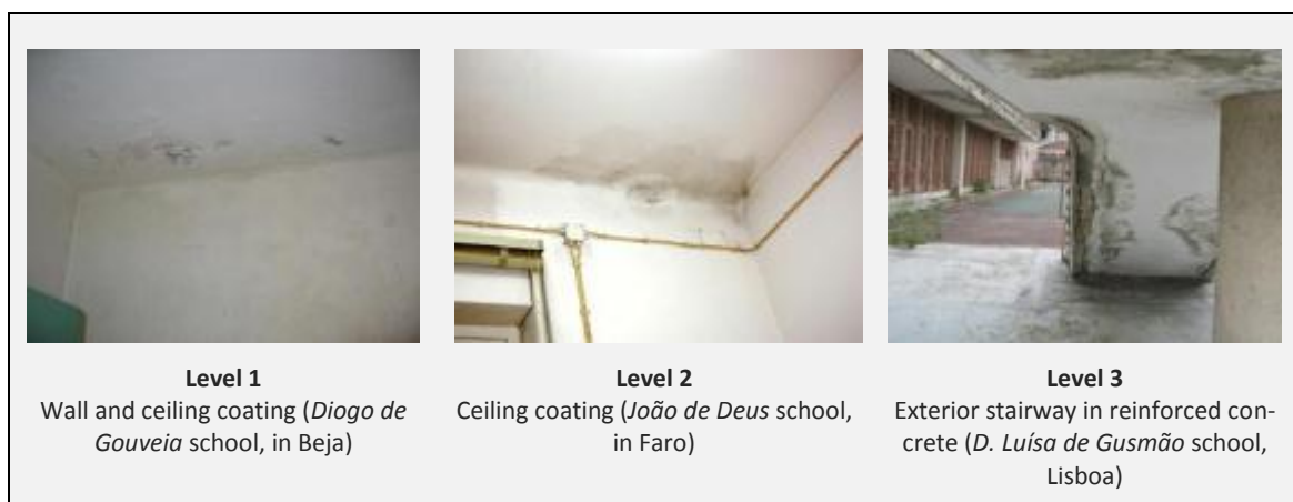
Fig. 13 - Example of a comparative visual evaluation for the A3 defect (discolorations or stains).
