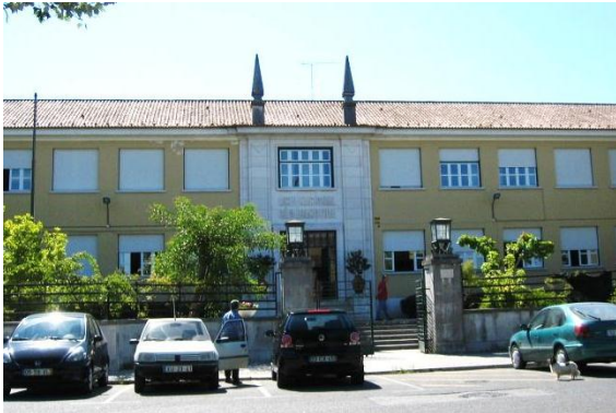
Fig. 9 - Main entrance of the Sá da Bandeira school, in Santarém (Branco et al 2008b).
